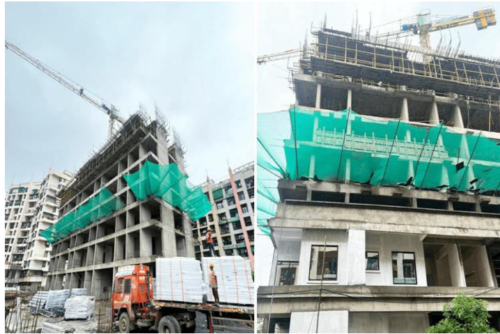
Figure 2: Two views of a multi-storey reinforced-concrete residential building under construction, showing slab/formwork activity, green safety netting, scaffolding, a tower crane, and on-site material handling
